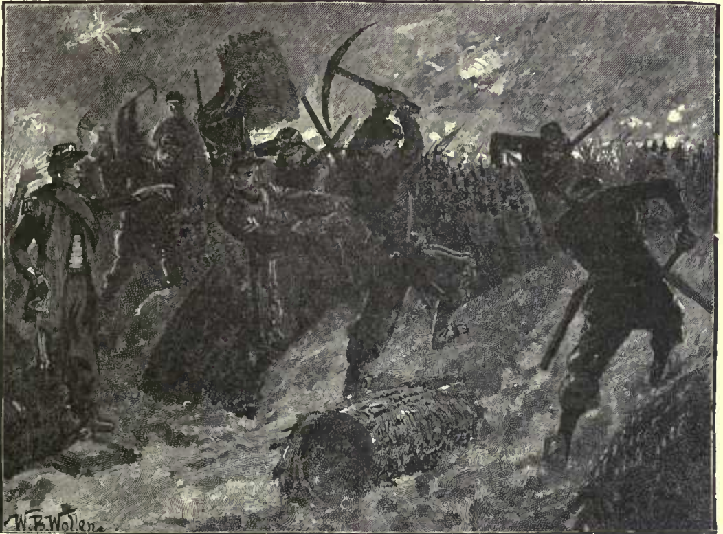
SAPPERS DESTROYING THE RUSSIAN TRENCHES. (See p. 99.)
